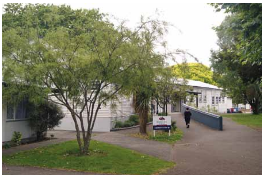
Whitiara School bathes under an extensive canopy of bright green trees
